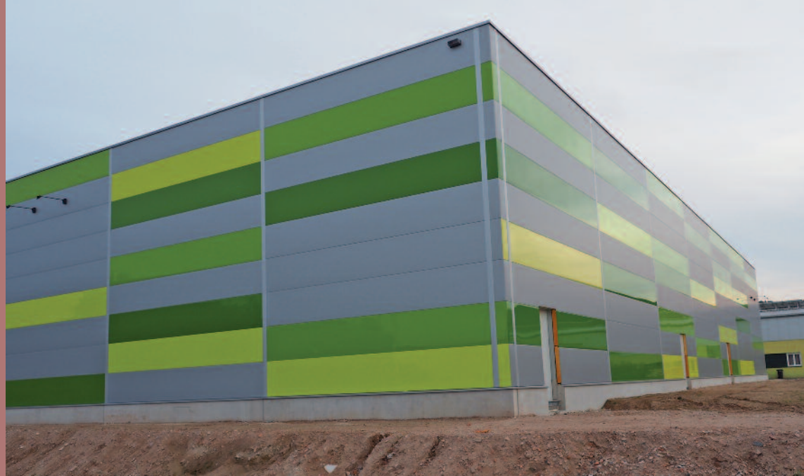
Die neue Kühlhalle in Spalt The new cold store in Spalt
